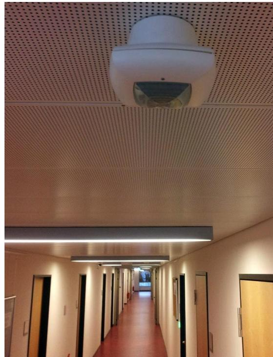
Figure 3. Siemens UP258/21 presence sensor in the 3<sup>rd</sup> floor of the office building under investigation. Sensors of this type are installed approx. every 8 meters in corridors and in some rooms.
